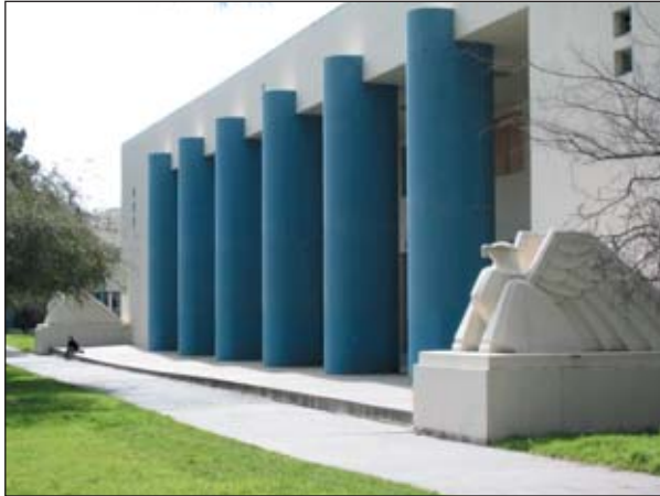
The former Bachelors Enlisted Men's Quarters could be adapted for work/live uses.
