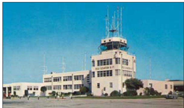
Two workshops were held in the former Flight Control Tower at Alameda Point.
