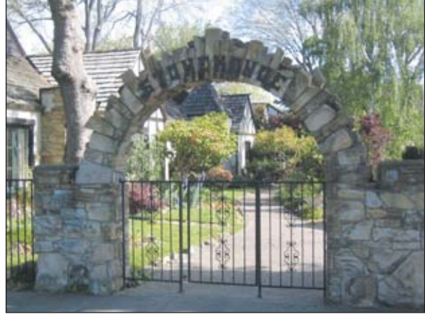
The Stonehenge on Santa Clara Avenue is an example of "mews housing".
